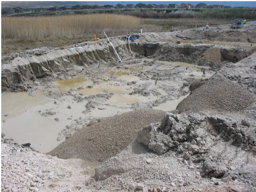
Figure 4-4. Excavation for Wall Embedment and Drainage Layer
